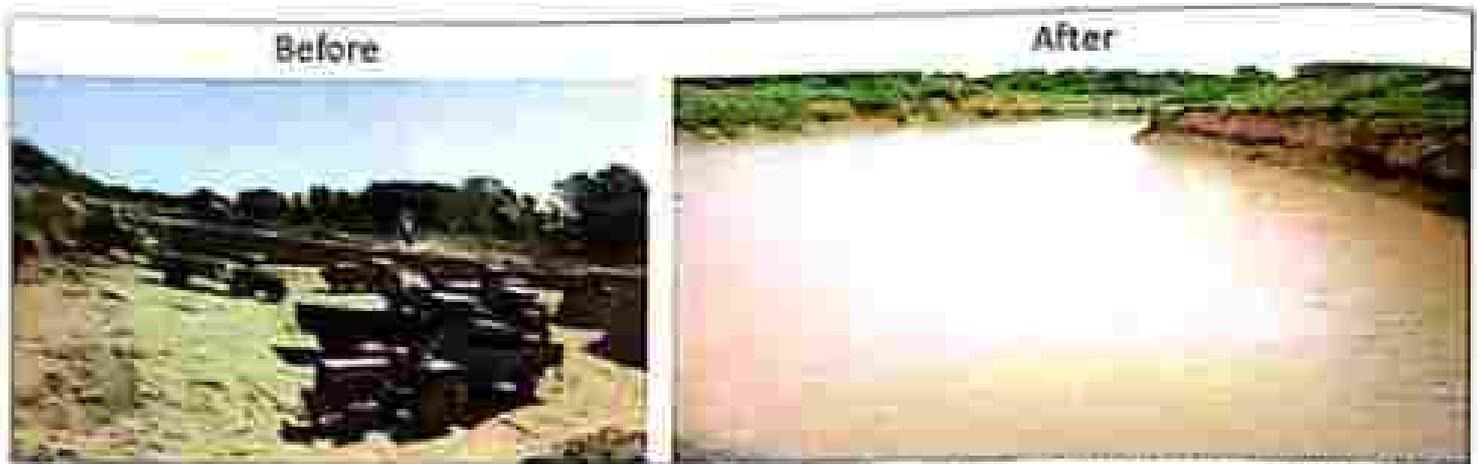
Figure 9: Before - after images of water conservation work in Ranaj village, Barakalatha. Increase in storage capacity by 1 lakh cubic feet.
